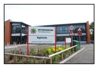
The steel framed structure was clad with standing seam roofing and a mixture of clay and aluminium wall cladding.
